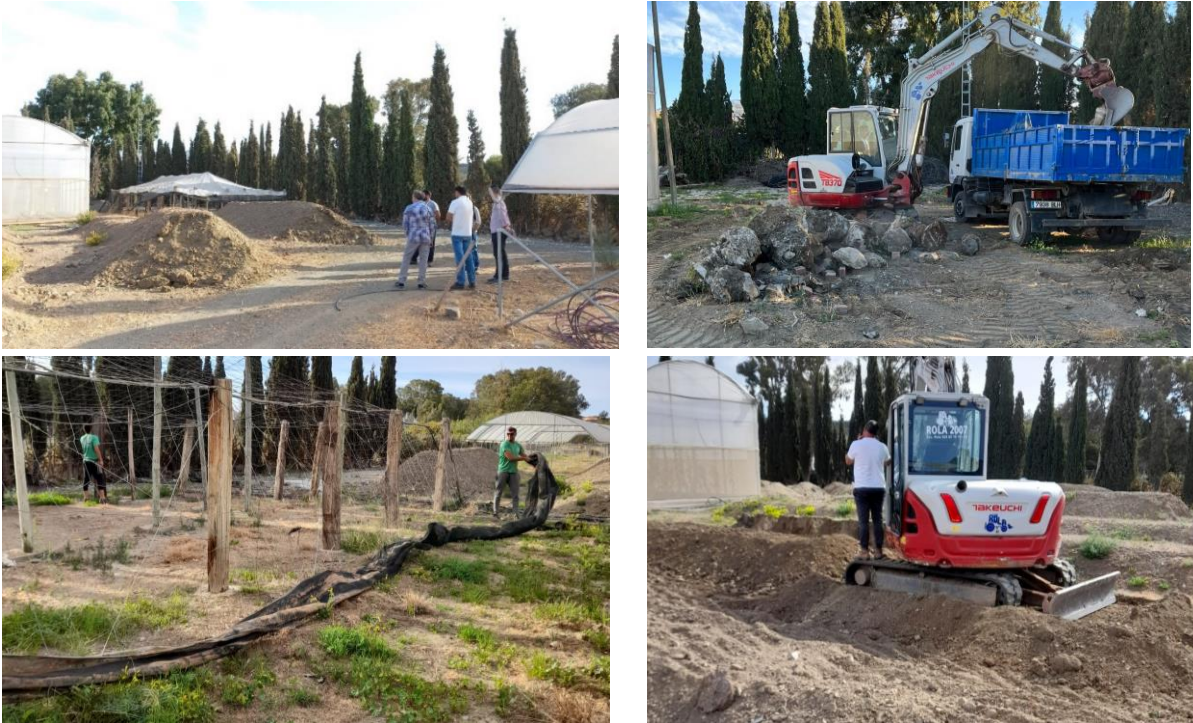
Figure 23. Test site construction and adaptation works.
